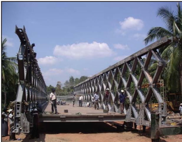
Fig. 11: Enacting temporary bridges
