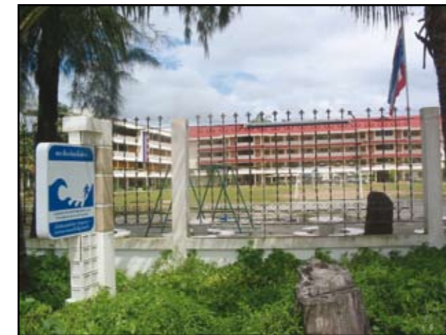
Fig. 7: Rebuilt School at Kamala.
