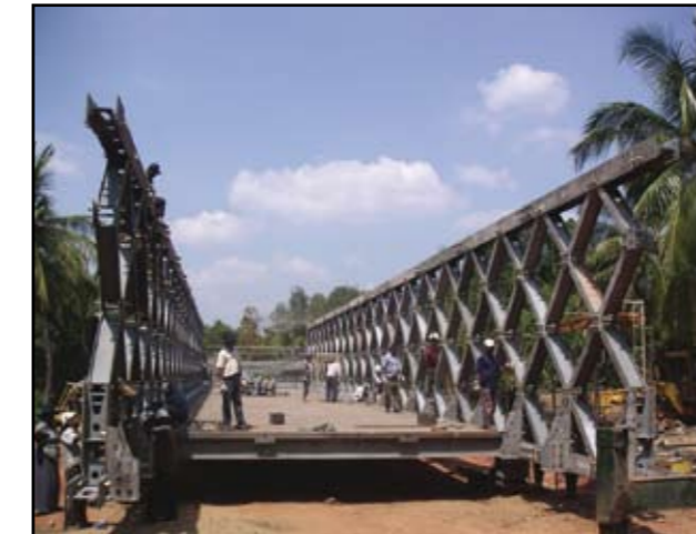
Fig. 11: Enacting temporary bridges
